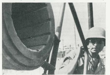
Close-up muzzle view showing the deep grooves into which shell splines fit.
